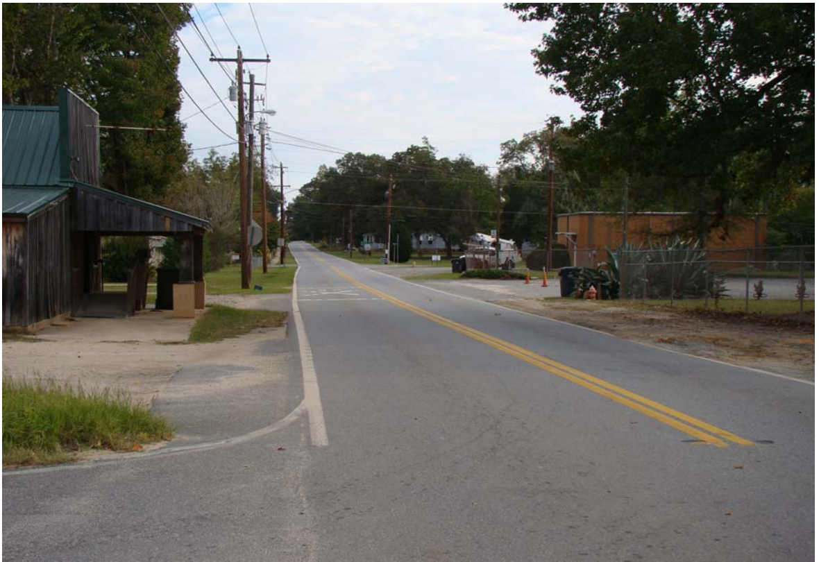
Photo 8: Lack of sidewalk connectivity into residential areas.
