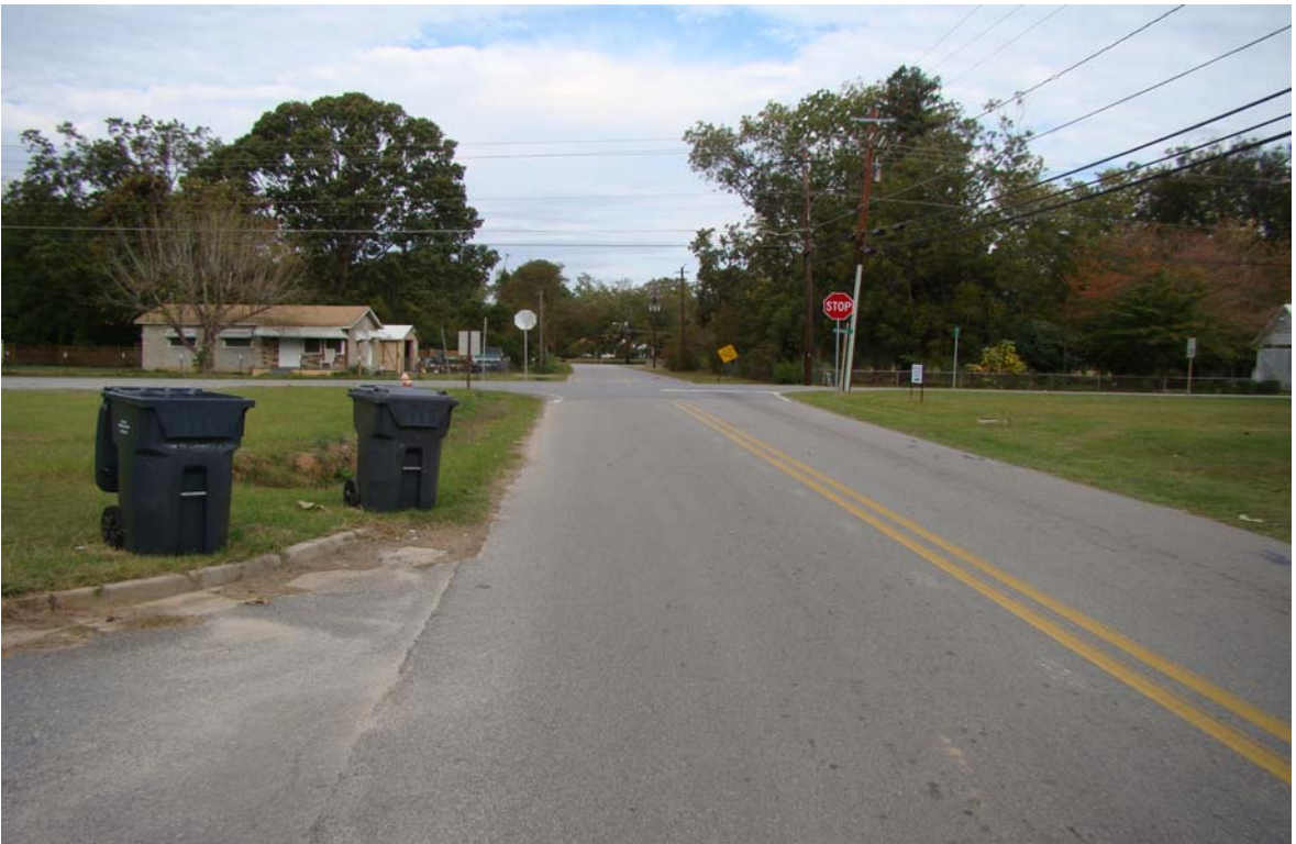
Photo 12: No sidewalk connectivity.
