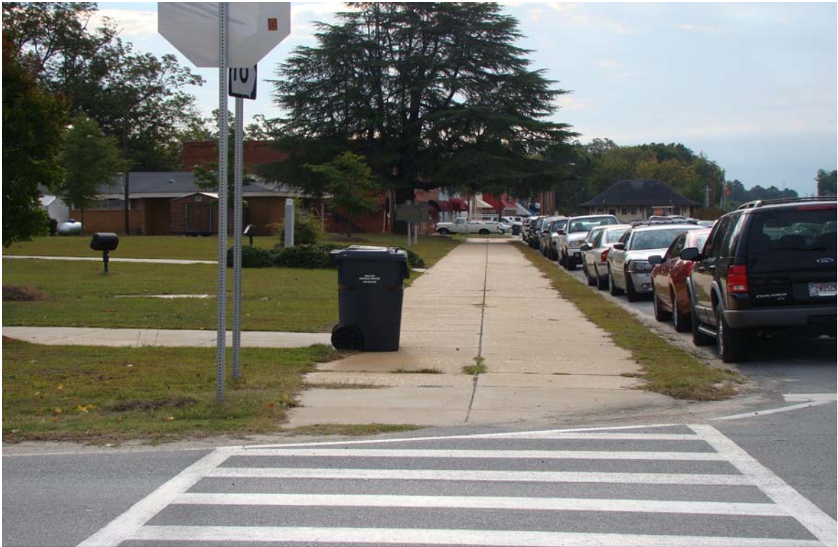
Photo 10: Sidewalk and crosswalk in front of Twiggs County Courthouse.
