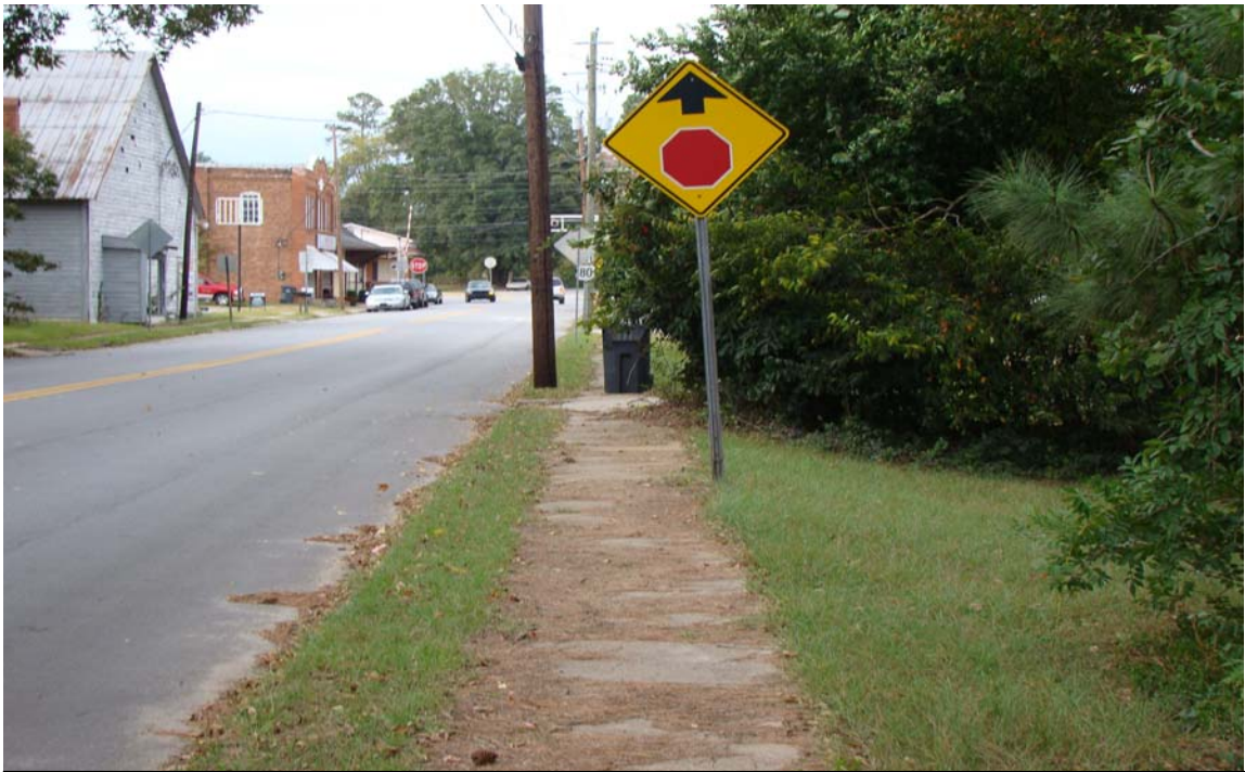
Photo 4: Poorly maintained sidewalk with obstructions.
